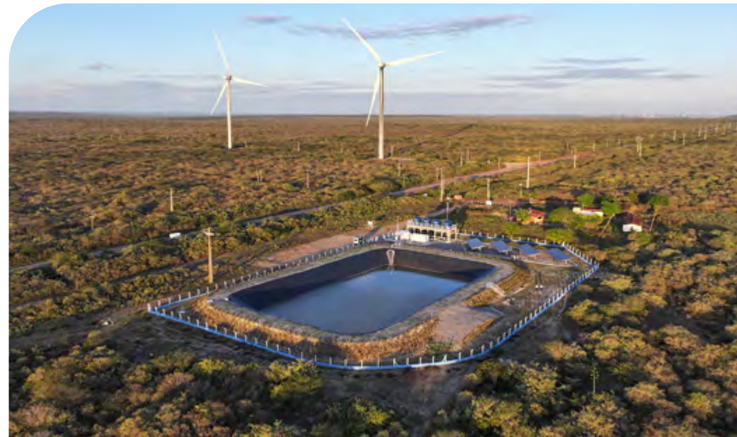
Water desalination plant built in the countryside of Rio Grande do Norte.
